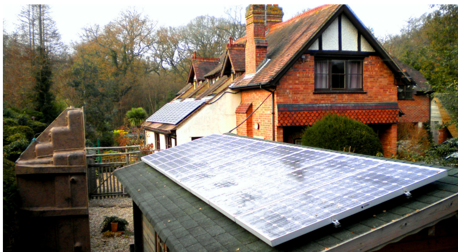
A 3.3 kWp installation consisting of one string with 18 modules that spreads across two roofs with two different slopes: 25° and 40°. The string is connected to a SolarEdge SE3300 inverter.
